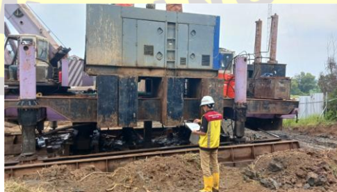
Gambar 67 Monitoring pekerjaan alat HSPD
