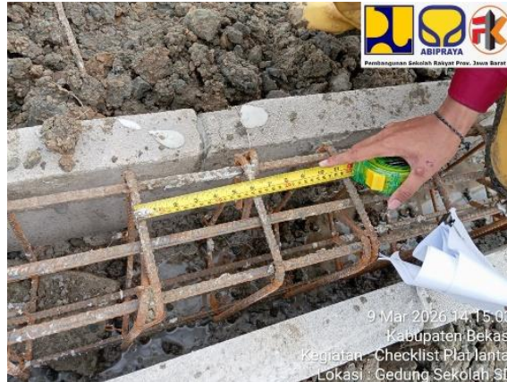
Gambar 49 Checklist pembesian tie beam
