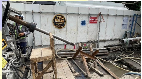
Dokumentasi Joint Survey Fist Pipe Jacking
