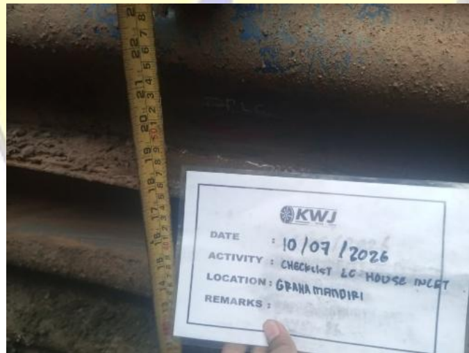
Gambar 3. 29 Checklist Rebar Lean concrete House Inlet Sumber: Penulis (2026)
