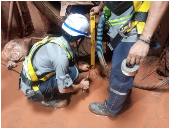
Gambar 3. 38 Marking Manhole
