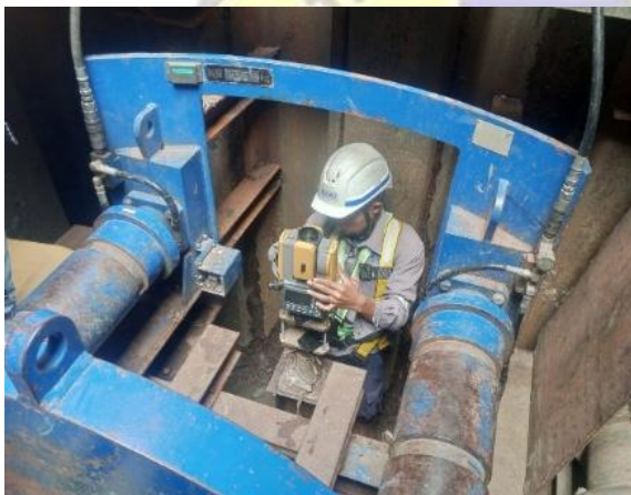
Gambar 3. 31 Setting Total Station Sumber: Penulis (2026)
