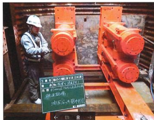
Gambar 2. 26 Instalasi Main Hydraulic Jack
