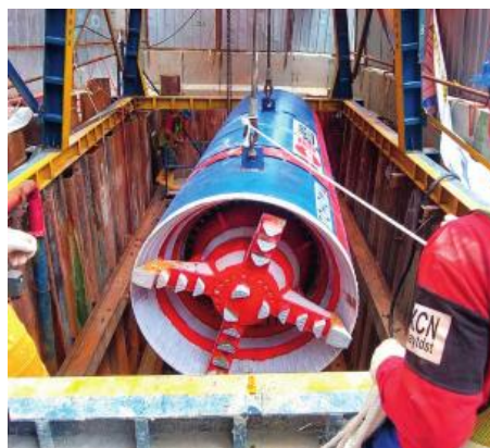
Gambar 2. 27 Cutter Head Sumber: TOHOMA (2017)
