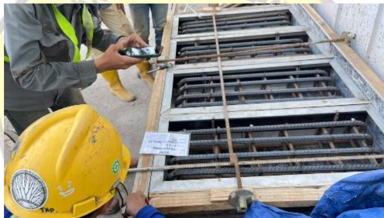
Gambar 3. 30 Checklist Rebar Cover Diversion Chamber Sumber: Penulis (2026)
