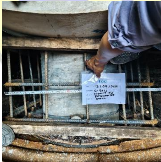
Gambar 3. 28 Checklist Rebar Protection Pipe
