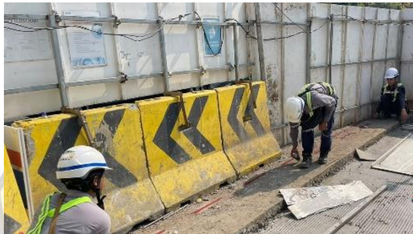
Gambar 3. 36 Marking Aspal
