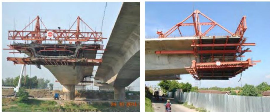
Gambar 1. 3 Metode Balanced Cantilever
