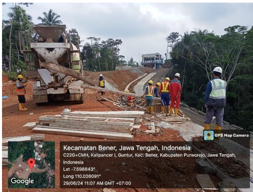
Gambar 3. 16 Truck mixer kapasitas 5 m 3
