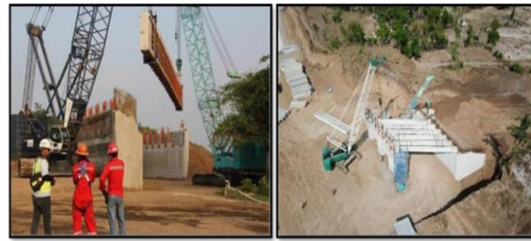
Gambar 3 Erection Girder
