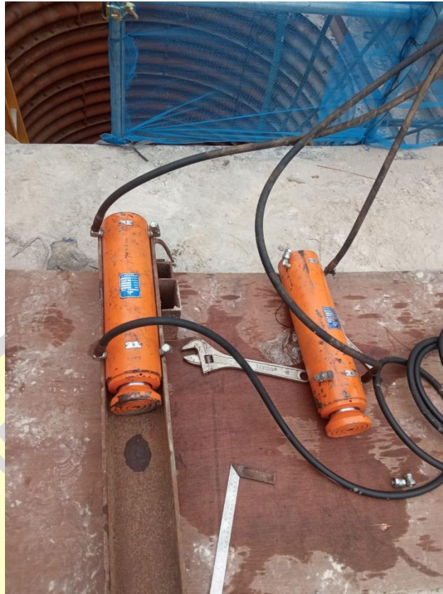
Gambar 5. 25 Instal hydraulic jack
